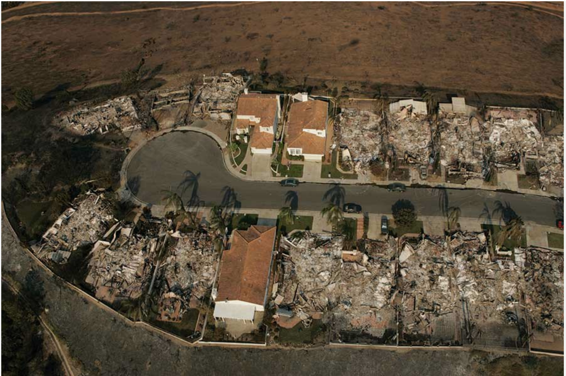
These three ICF homes in San Bernardino were the only survivors in the neighborhood after a devastating 2007 wildfire.
